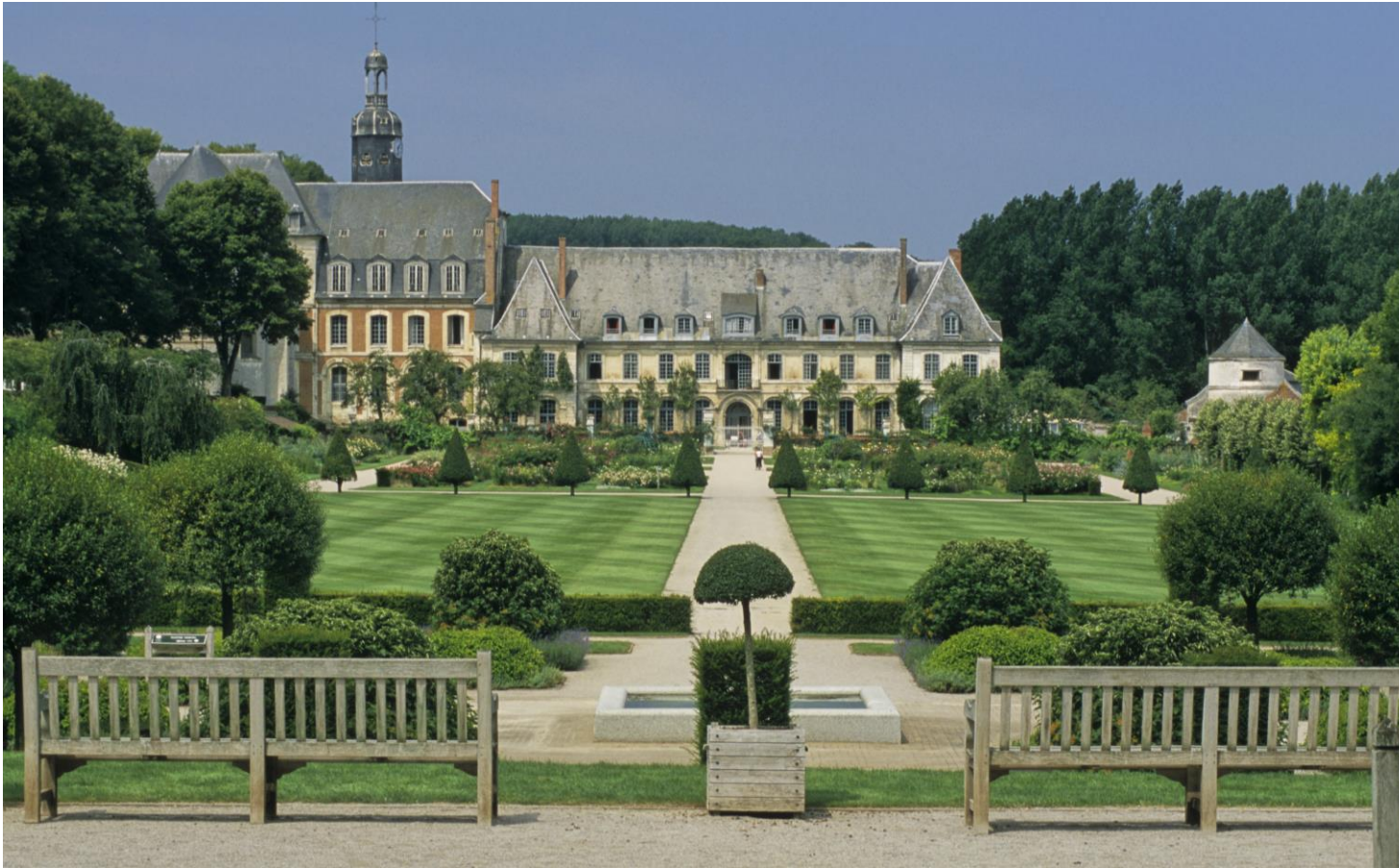
Front view from the gardens of the East facade
